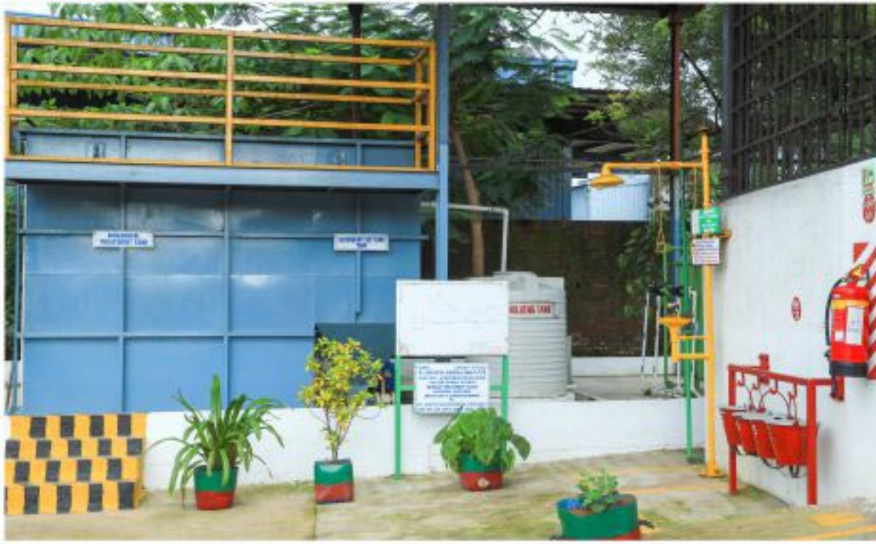
Sewage Treatment Plant
